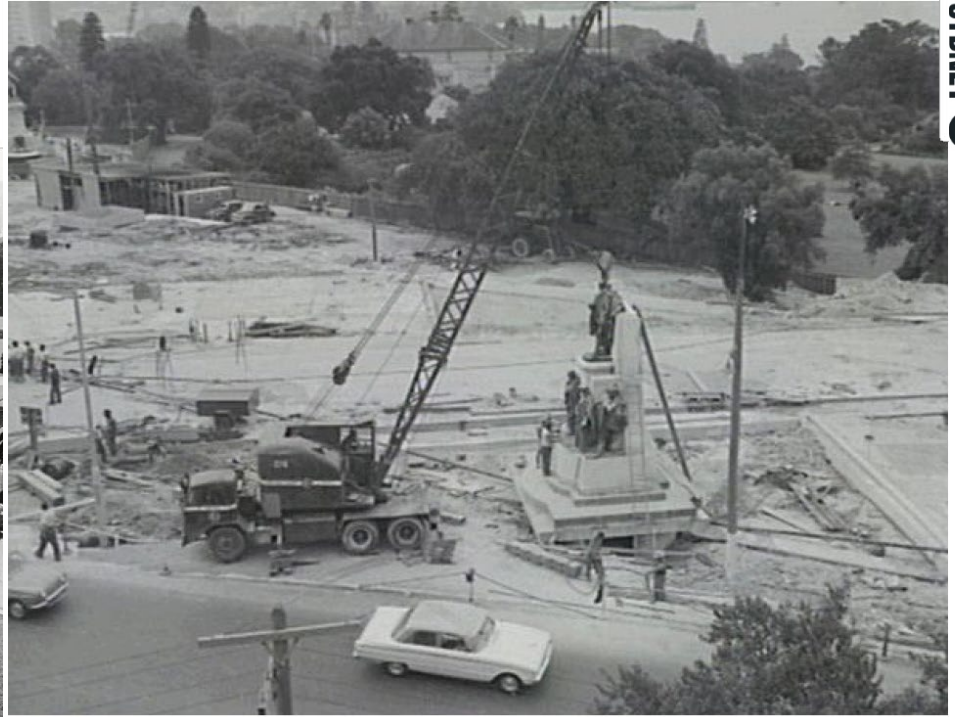
Cahill Expressway construction, repositioning Shakespeare Memorial Sculpture, Sydney, 1962, City of Sydney Archives
